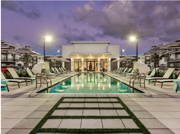
The MID, with 230 residential units and 10 retail units, in Lake Worth Beach
